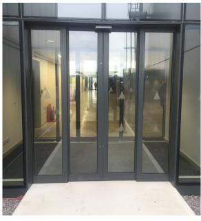
The Glide T allows for operation of telescopic doors.
